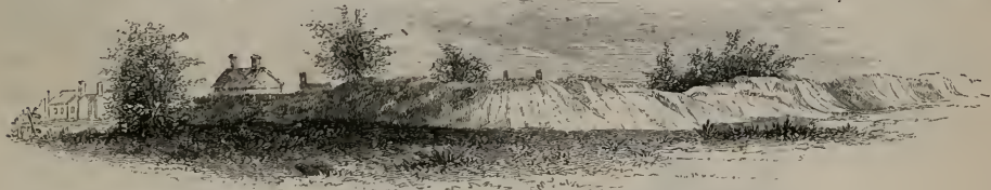
PRESENT APPEARANCE OF THE BRITISH WORKS AT YORKTOWN. 1
